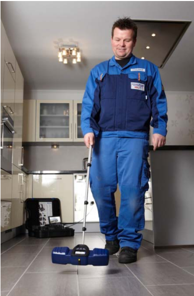
Fig. 11: Localizing the camera head underground
